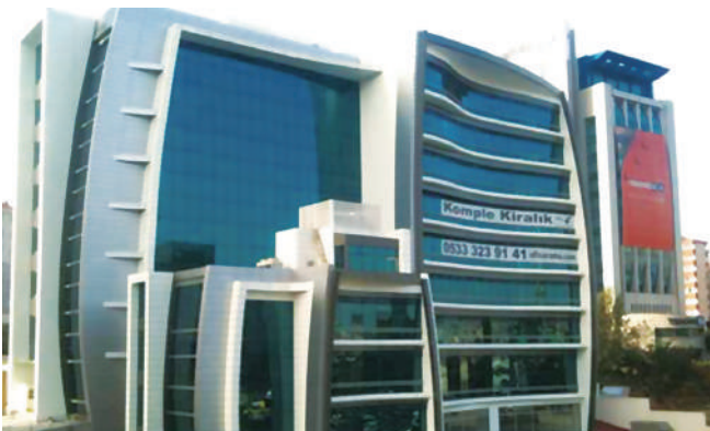
Office building in Istanbul, Turkey.
