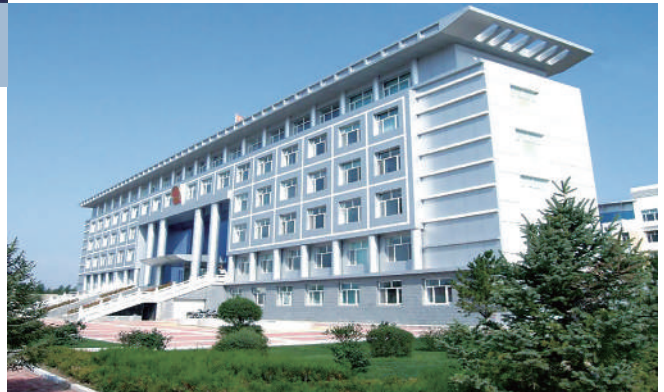
Government building in Inner Mongolia , China.
